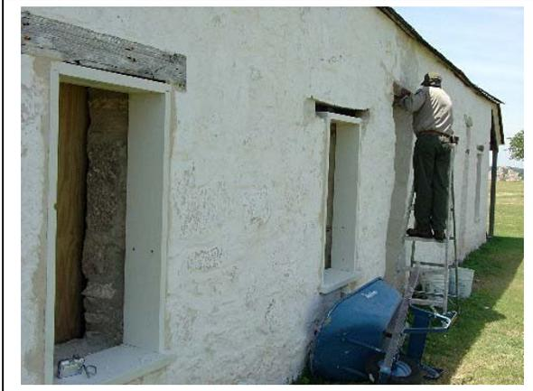
*Left: Ranger Ken Lester working on one of the headers for Officers Quarters No. 3. The windows were literally falling out and had to be rebuilt and fitted to the building.*
